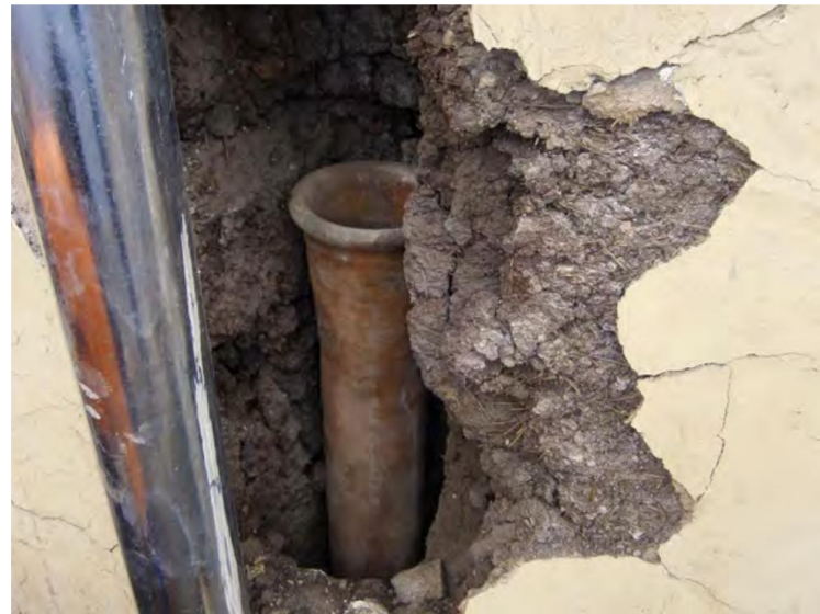
Replacement of defective piping at the Carvallo House (LA)
