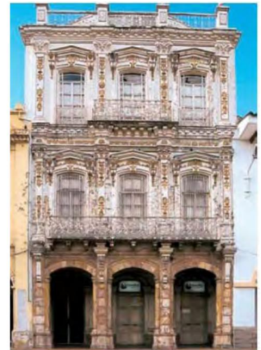
Facade of the Hortensia Mata Passage (Regional Government of Andalusia, 2007, Architecture Guide, Cuenca, Ecuador)
