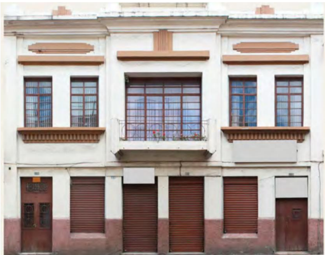
Facade. (Source: University of Azuay. 2013. The built heritage in Cuenca. Architectural photogrammetry)
