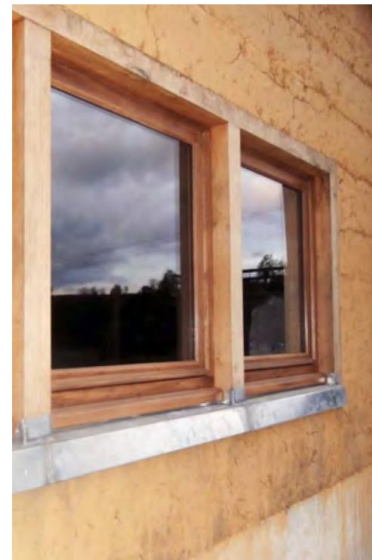
Extended windowsill with metal element (ES)
