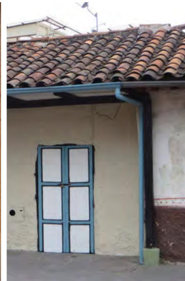
Downpipe outside the wall (IS)
