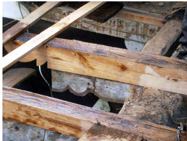
Extension of the eaves with new joists (LA)
