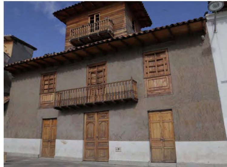
The same wall after plaster repair (AR)
